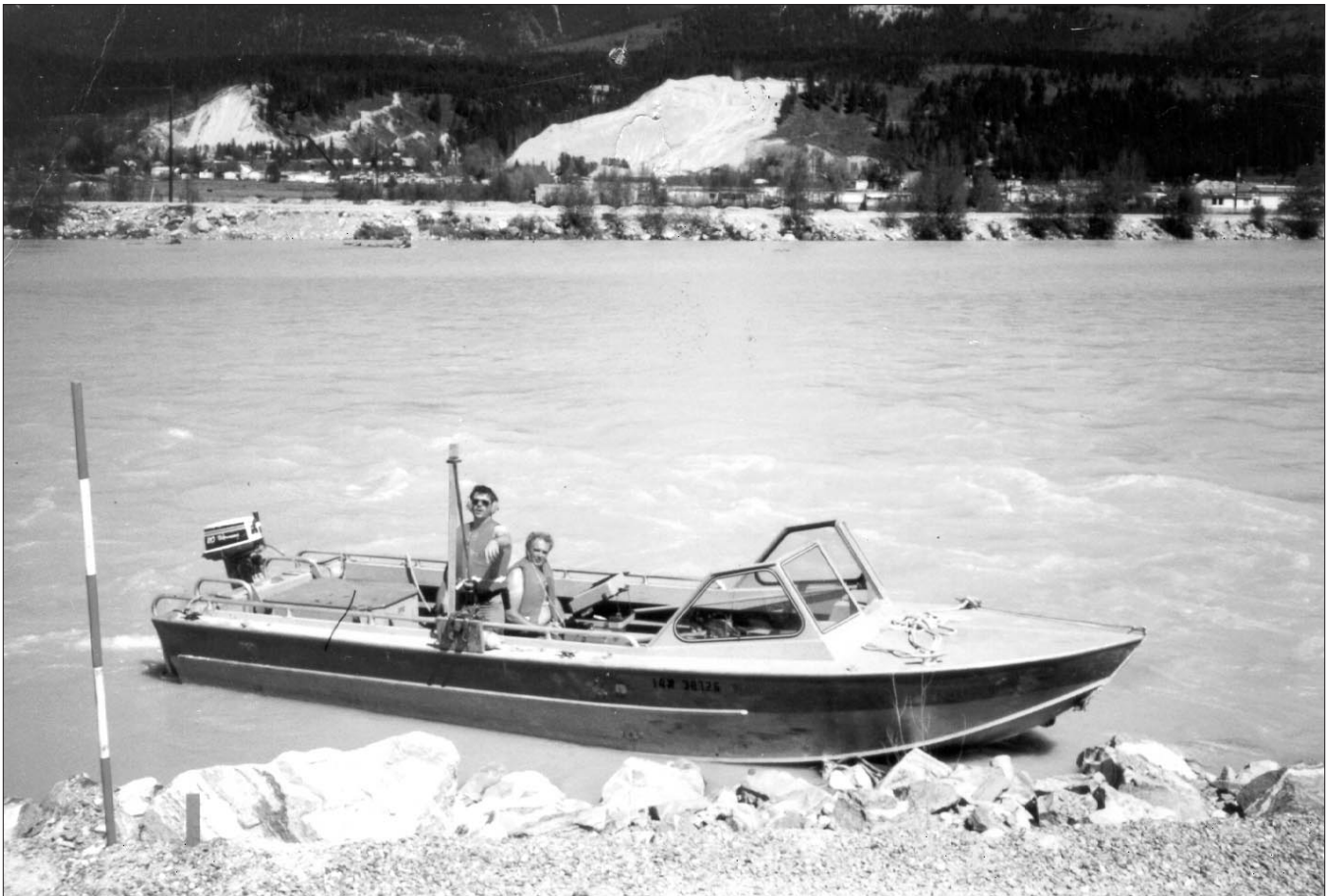
Inspections by Boat
